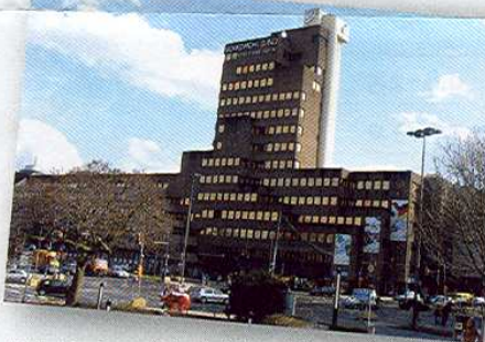
This Dortmund demolition job created a major challenge for the three German contractors tasked with its demolition
