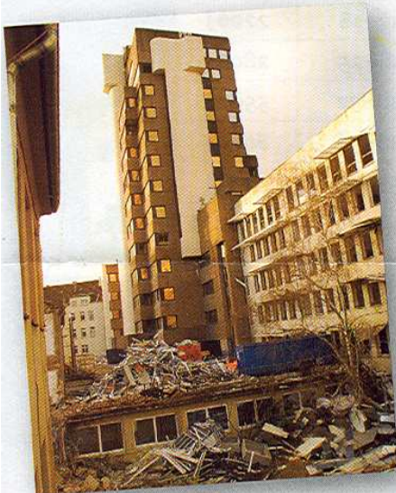
Ready for blowdown, Soft strip has been carried out, surrounding lower associated structures cleared and charges are set
